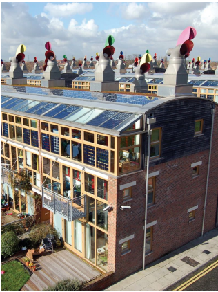
BedZED in Wallington
